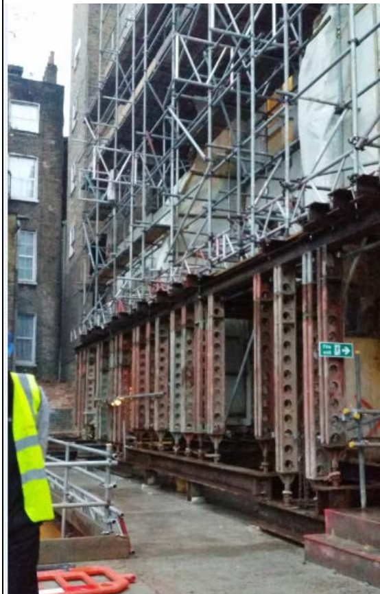
Rear Elevation (under construction)
